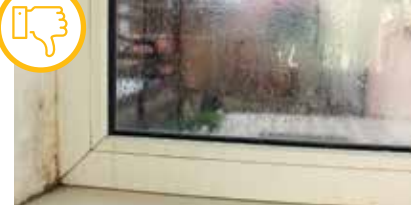
Uninsulated window with condensation.
