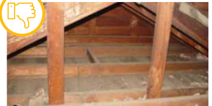
Attic not prepped or insulated. Courtesy of U.S. Department of Energy
