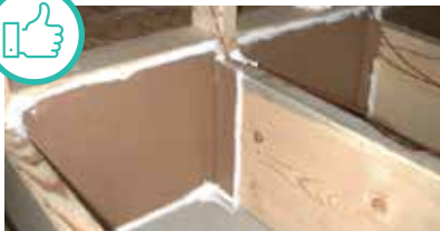
Floor joists under kneewall (blocked with rigid material and sealed with caulk). Courtesy of U.S. Department of Energy
