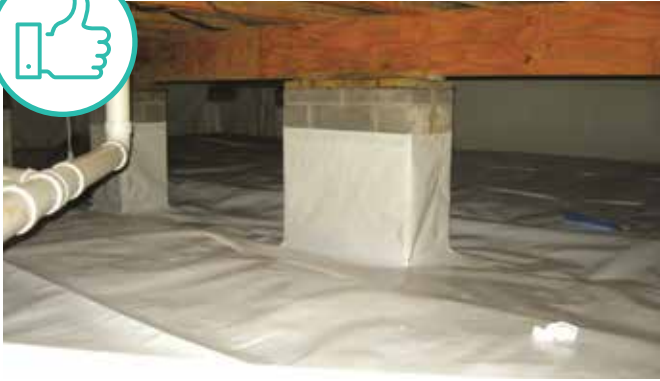
Seams overlap, laps up foundation.
