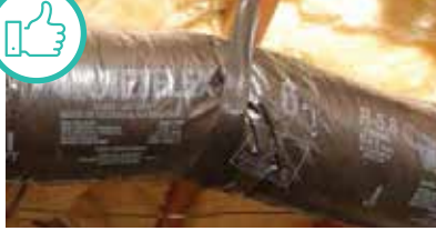
Duct properly supported.
