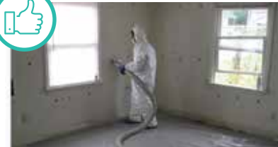
Insulating brick or stucco wall from interior.
