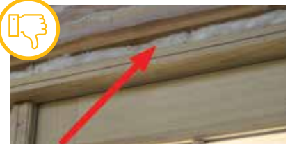
Incomplete seal around newly installed window.
