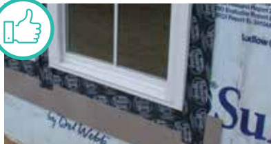
Proper flashing window to weather barrier.
