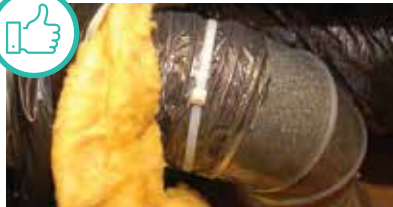
Flex duct is properly fastened to metal duct with mechanically tightened strap.
