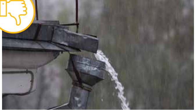
Rusting, disconnected downspout.
