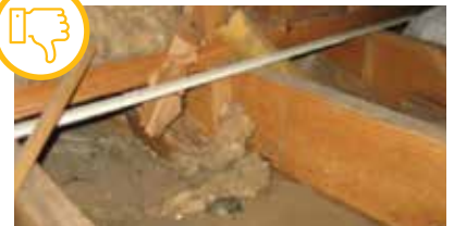
Floor joists under kneewall (not blocked with rigid material and unsealed). Courtesy of U.S. Department of Energy
