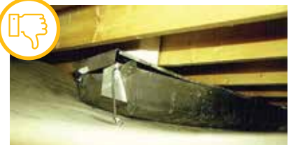
Uninsulated belly with duct leakage.
