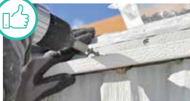
Edge of roof secured and gutter re-attached.
