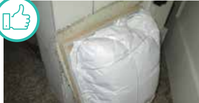
Crawl hatch insulated and weatherstripped.
