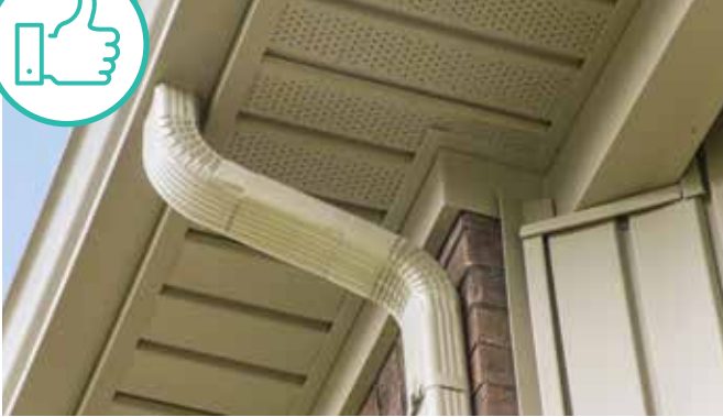
Inspect all downspouts for proper connection.
