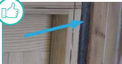
Backer rod and caulk complete seal around window frame.
