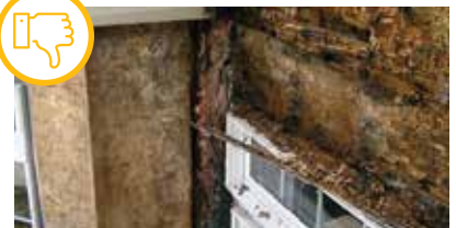
Improperly flashed door has structural damage due to water penetration. Courtesy of U.S. Department of Energy
