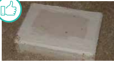
Non-IC fixture with drywall shield (hat).
