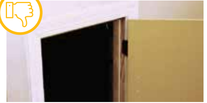
Uninsulated, not weatherstripped. Courtesy of Advanced Energy
