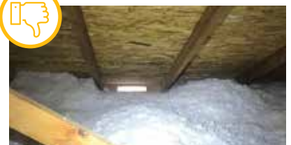
Roof-to-wall heel uninsulated. Courtesy of Advanced Energy
