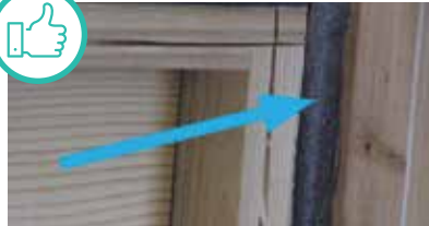
Closed-cell foam seals the gap. Courtesy of U.S. Department of Energy
