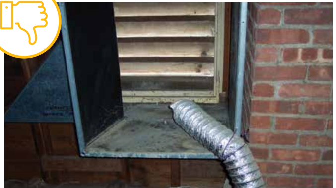
Not insulated, vented to exterior or properly supported.
