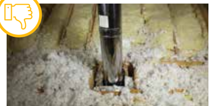
Unsealed penetration (heat-producing).
