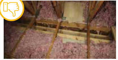
Open/unsealed chase or cavity.
