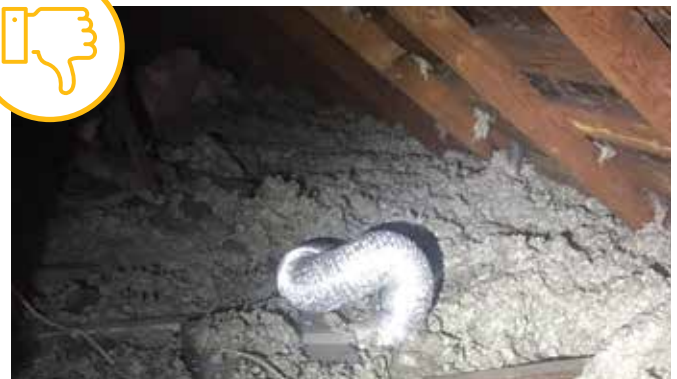
Poorly ducted, vented to attic.
