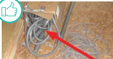
Backer rod for sealing around window.
