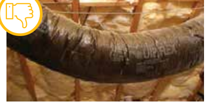
Duct is not properly supported.
