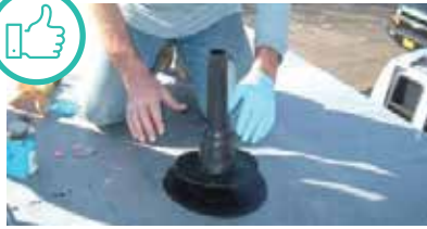
Roof penetration properly sealed.
