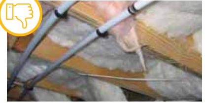
Insulation does not fill cavity and not properly supported.
