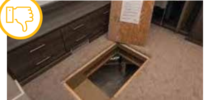
Crawl hatch NOT insulated or weatherstripped.
