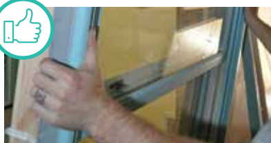
Proper fit window, level, and sealed.
