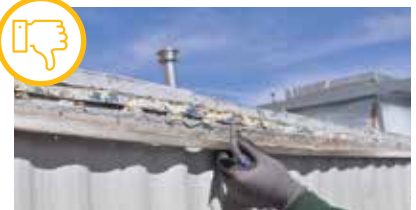
Gutter not properly attached, potential leaks at roof edge.
