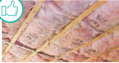
Insulation fills cavity, properly supported.
