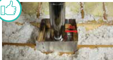
Sealed penetration (heat-producing).
