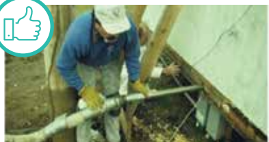
Insulating belly from edge fill method.
