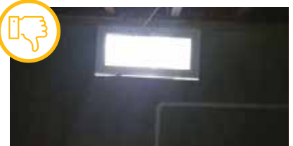
Window install not sealed, improperly fit.
