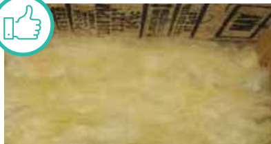
Insulation in full contact with floor.
