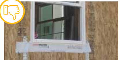
Improperly flashed window.
