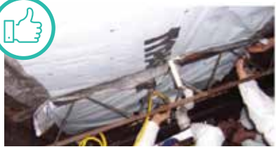
Repaired and supported belly material.
