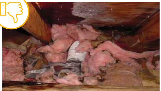
Interior moisture source not corrected. This problem is due to an unvented fan.
