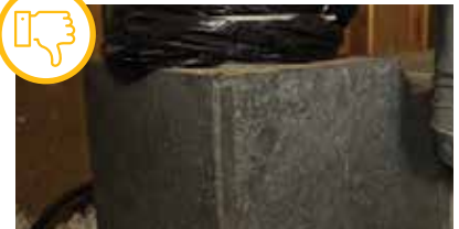
Unsealed duct plenum.
