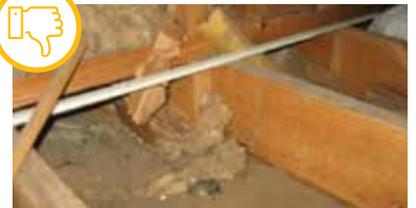
**Floor joists under kneewall (not blocked with rigid material and unsealed).**
