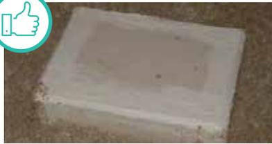
**Non-IC fixture with drywall shield (hat).**
