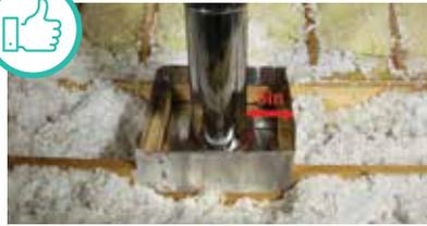
**Sealed penetration (heat-producing).**
