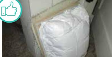
**Crawl hatch insulated and weatherstripped.**
