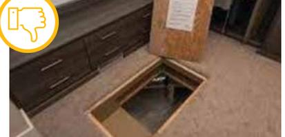
**Crawl hatch NOT insulated or weatherstripped.**
