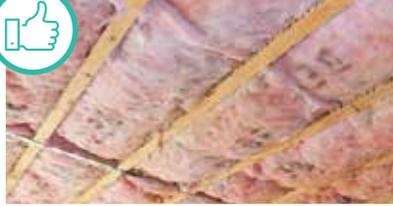
**Insulation fills cavity, properly supported.**
