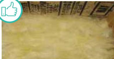
**Insulation in full contact with floor.**
