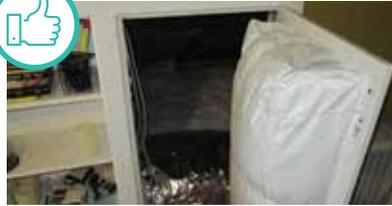
**Weatherstripped and insulated hatch.**
