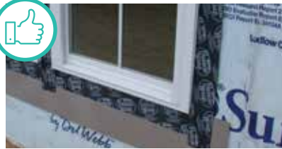
Proper flashing window to weather barrier. Courtesy of U.S. Department of Energy
