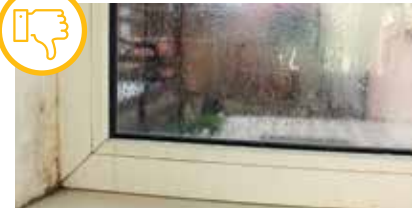
Uninsulated window with condensation.
