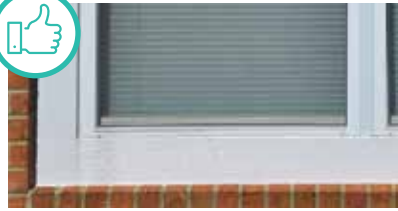
Double-paned window, installed with proper flashing.
