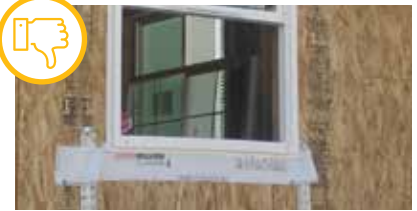
Improperly flashed window. Courtesy of U.S. Department of Energy
