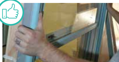
Proper fit window, level, and sealed. Courtesy of Santa Fe Community College
