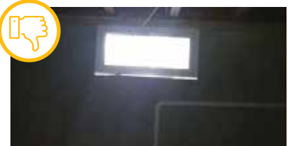
Window install not sealed, improperly fit. Courtesy of U.S. Department of Energy
