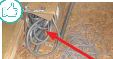
Backer rod for sealing around window. Courtesy of U.S. Department of Energy
