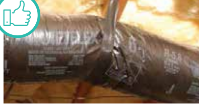
Duct properly supported. Courtesy of Advanced Energy
