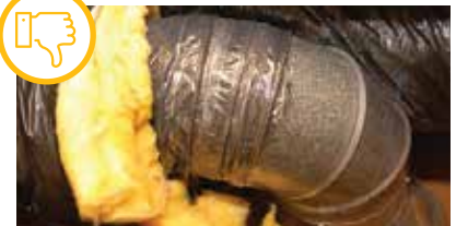
Flex duct is not mechanically fastened to metal duct. Courtesy of Advanced Energy
