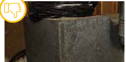
Unsealed duct plenum. Courtesy of Advanced Energy
