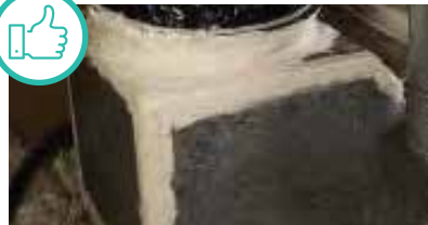
Plenum sealed with water based, fiber embedded duct sealing mastic. Courtesy of Advanced Energy
