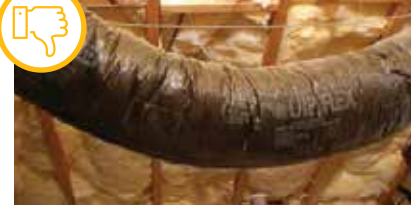
Duct is not properly supported. Courtesy of Advanced Energy
