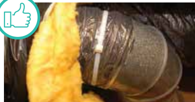
Flex duct is properly fastened to metal duct with mechanically tightened strap. Courtesy of Advanced Energy
