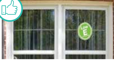
Single-paned aluminum window with well-fit storm window.
