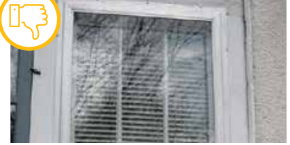
Single-paned aluminum window with no storm or low-e protection.
