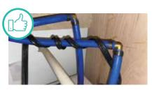
When insulation is not enough, use heat tape to prevent freezing.
