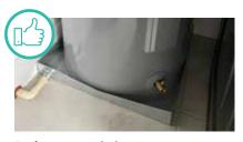
Drain pans can help prevent messes and water damage.
